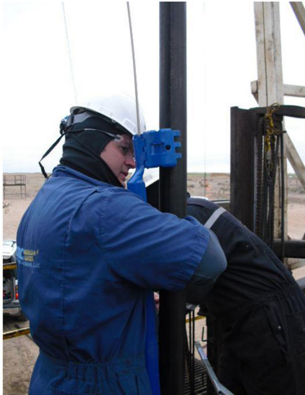
Figure 20. Install clamp on tubing and use a clamp closing tool to close clamp.
